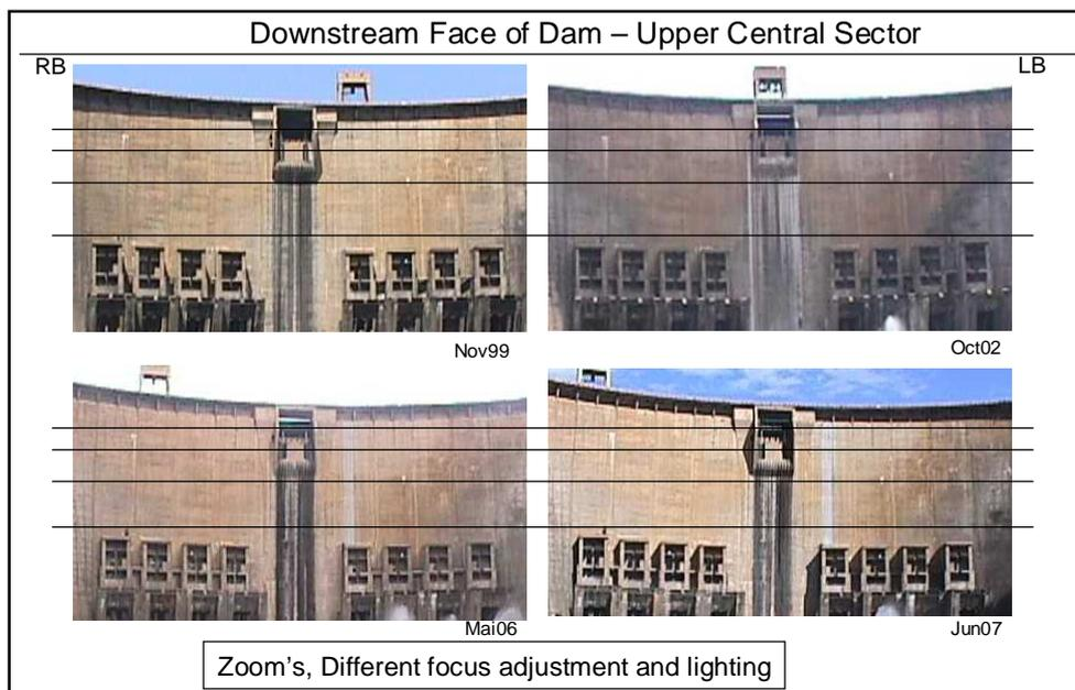
Fig. 4 – Historical sequence of photographs from the downstream face of the dam
