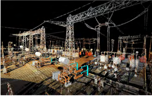
Figure 2: Hydropower substation 3D surveying and modeling of the Cahora Bassa dam in Mozambique. Point clouds have been coloured by projecting the photogrammetrically processed acquired images.
